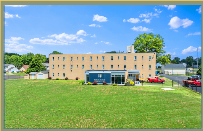
External View of the Dorm Building
